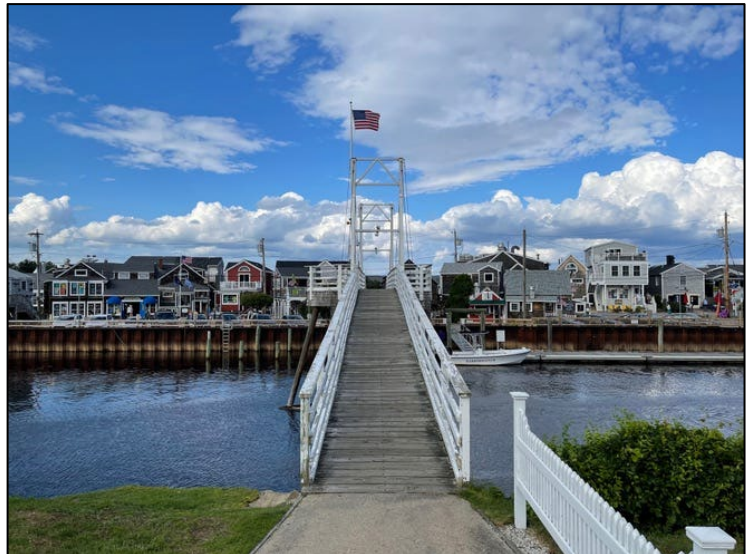
Photo 4 Perkins Cove Bridge
