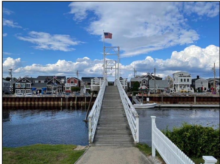
Photo 4 Perkins Cove Bridge
